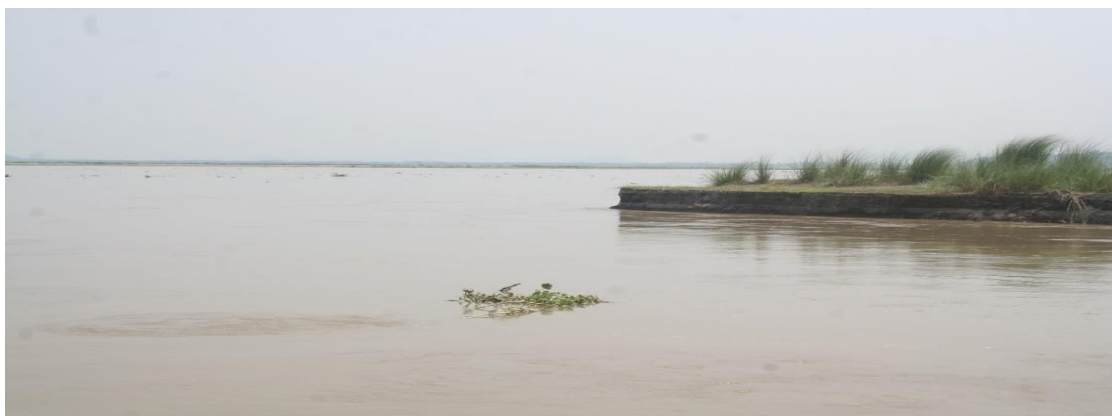
Erosion by Brahmaputra River in Maleghar Gram Panchayat
