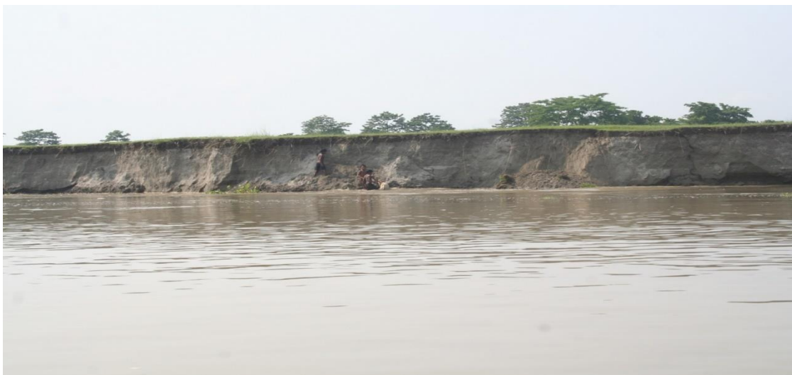
The picture shows erosion in Malegarh GP of Tapattary Block
