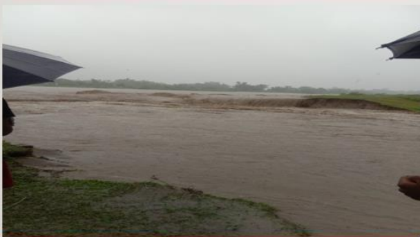
Brahmajan embankment breached, Chirang
